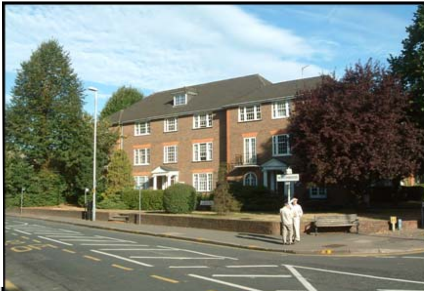
Greenhill Court, Dene Road, Northwood, HA6 2DB
